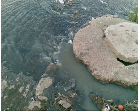
**Plate 4: An accidental burst sewer in Tassia estate where wastewater finds its way into Ngong River (Source: Author, 2013).**
