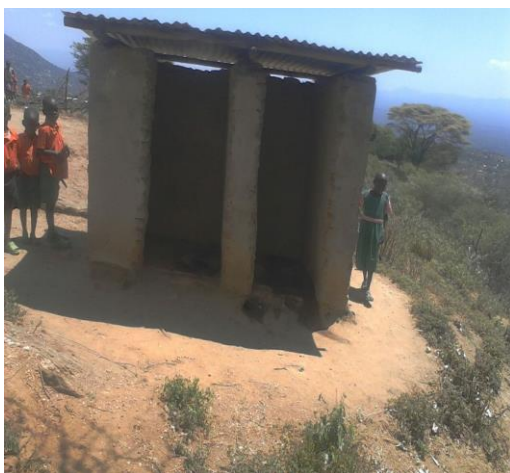
Plate 3: An ECDE School Latrine
