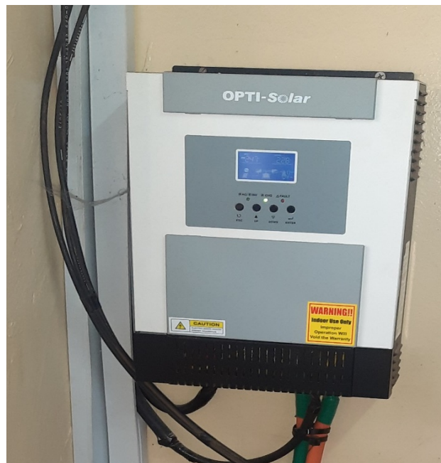
Figure 3.4: Picture of Integrated Inverter/Controller Unit.
