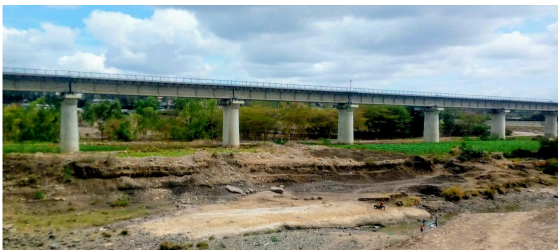
Figure 4.11 Standard Gauge Railway cutting across the Kitengela corridor.
