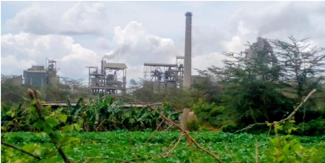
Figure 4.12 Cement factory constructed within the Kitengela corridor.
