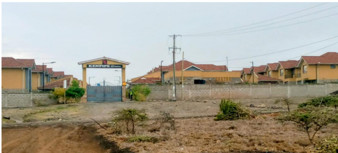
Figure 4.10 KenPipe Garden Hotel constructed within the Kitengela corridor.
