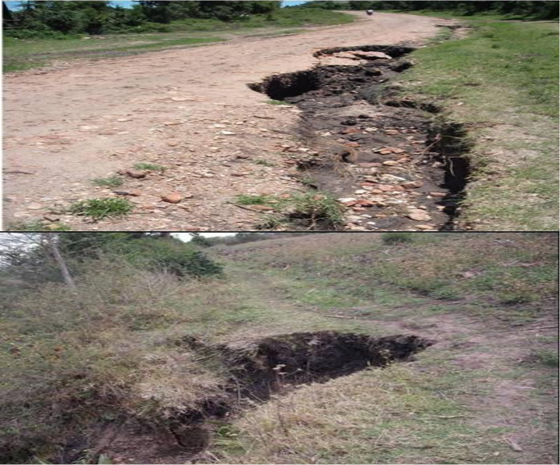
Plate 6.3: Part of Bomet-Sigor road (above) and eroded edge of a farm (below) damaged by erosion (Source: Author, 2010)
