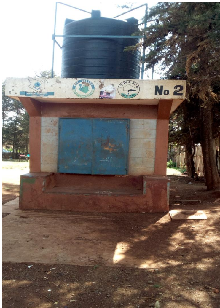
Plate 4. 2: Community Water Kiosk at Kariobangi Estate
