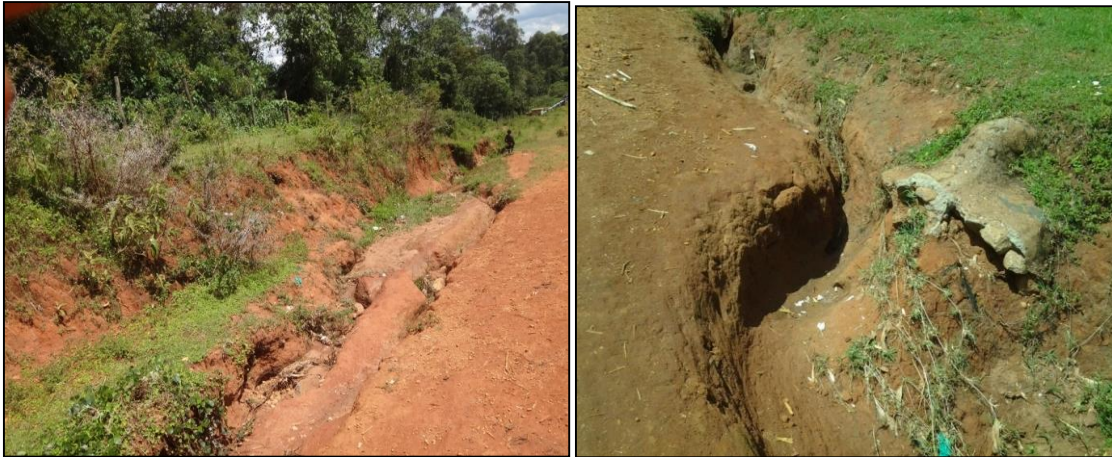
Figure 4.19: Gully erosion (left) and a failed scour check near Saiwa swamp (right). Author (Source 2013).
