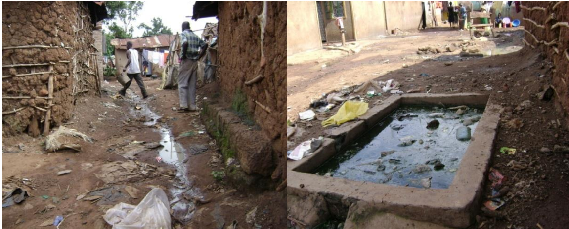
Plate 2: Site where there is no sewer line in operation in the Municipality
