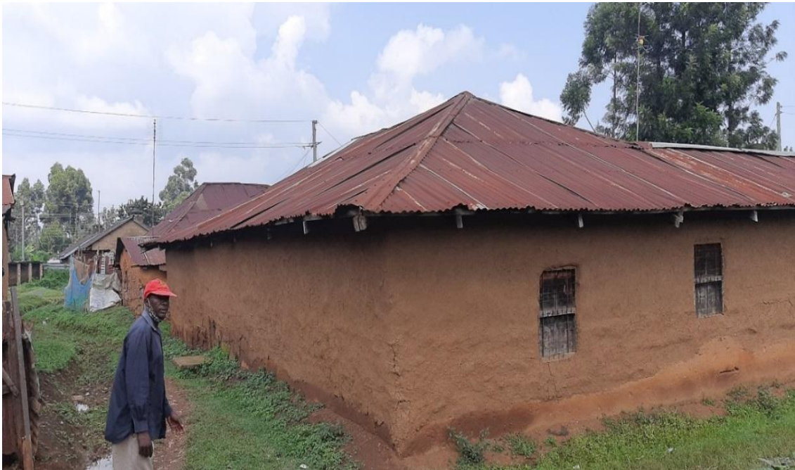
Plate 10: Roofs without gutters in Amalemba informal settlement.
