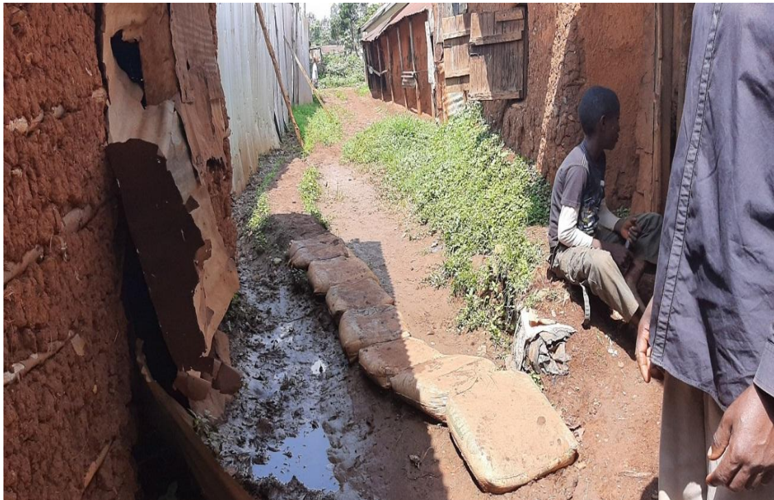
Plate 15: Cement bags filled with soil used to control runoff in Amalemba informal urban settlement.
