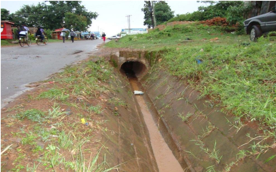
Plate 18: A Culvert in Amalemba informal urban settlement used to convey runoff.
