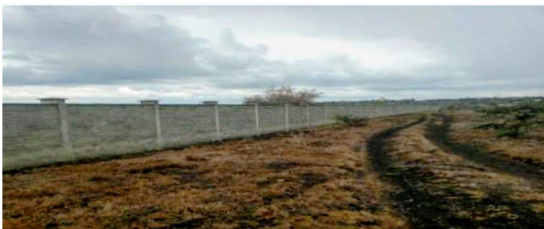
Figure 4.8 Wildlife-proof fencing for a private farm within the Kitengela migratory corridor
