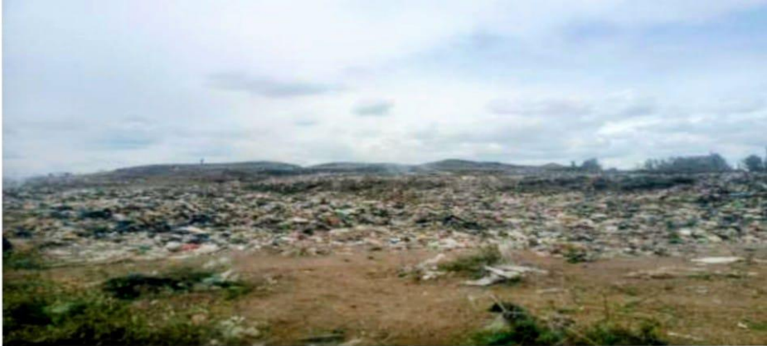
Figure 4.6 Kitengela dumping site located within the wildlife corridor.
