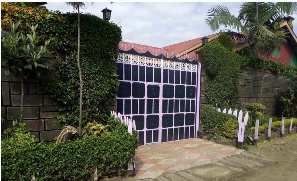
Plate 4.6: An Exterior Design that would Fit any Personality Colour Scheme Designed by KIDDG
