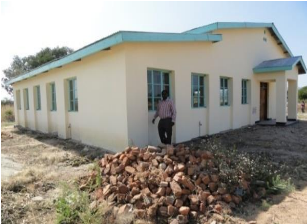
Plate 5.11: A dispensary built in Makifu village, Iringa using funds accrued from wildlife conservation. (Source: Author, 2012)
